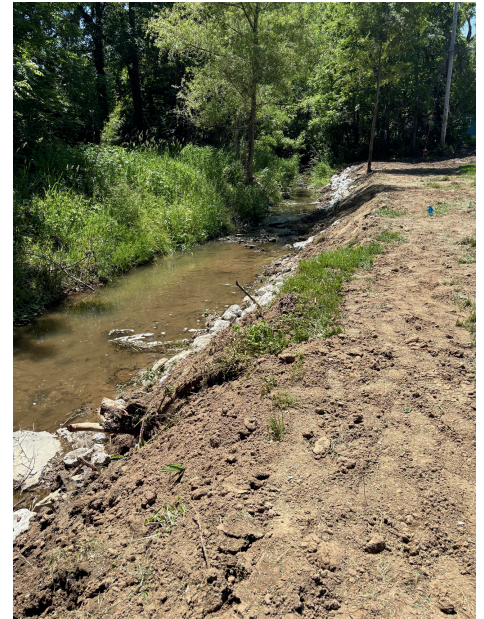
The recently finished streambank stabilization project in Andalusia, IL.
