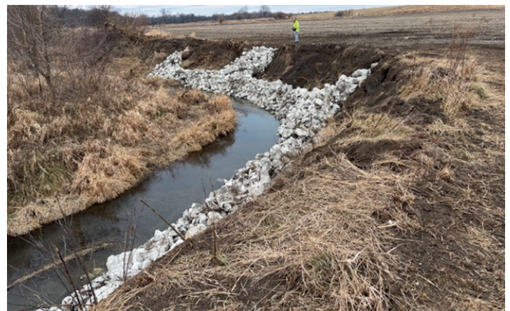
Streambank stabilization project on Mill Creek in Rock Island County.
